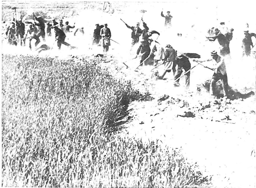
Commune members clearing away sand to make new fields.
